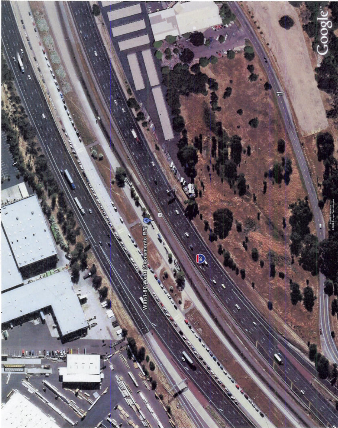
Watt West Light Rail
